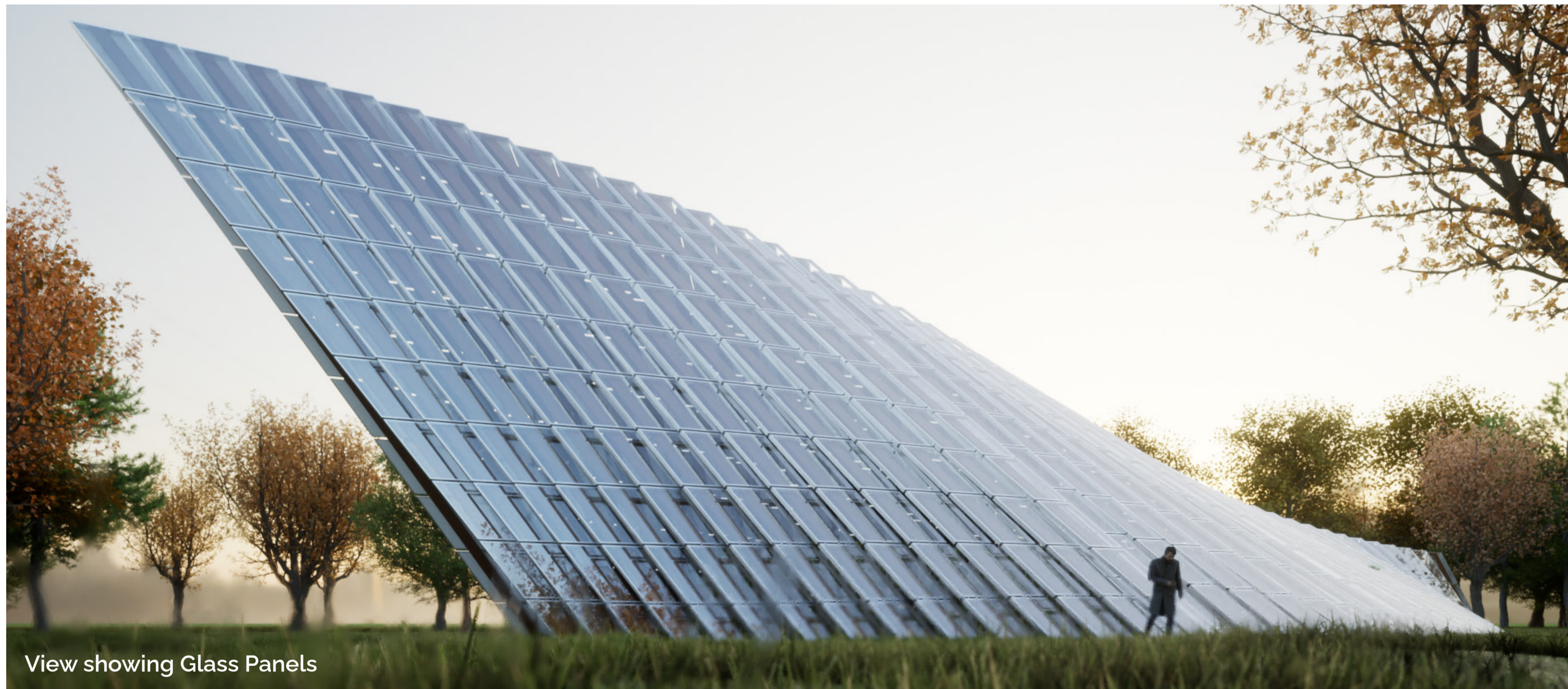
View showing Solar Panels
