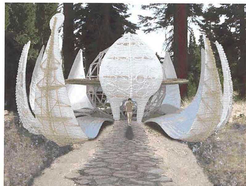
Figure 4: The entrance ramp to the building is 19 meters long at a 1:12 slope to accommodate physically challenged individuals and to be used as a solar exposure ramp for rolling the triple-solar-oven apparatus down the ramp into the sunlight. Luminescent pebble stones are placed between the circular tree slab ramp flooring—night lighting without electricity. Digital photo rendering by Yeyo Xral.
