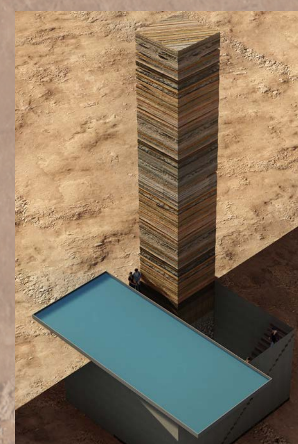
Cooled Indoor Room Roof Tray Collecting Rainwater
