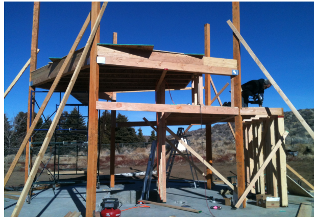
Central core area is constructed separate from the exterior walls.
