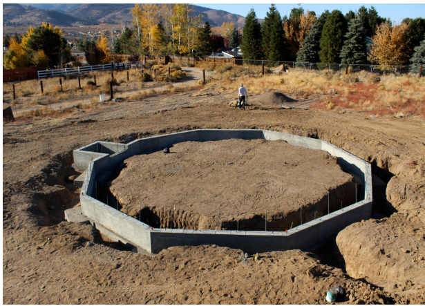
Compact decagon footprint means less ground area is impacted.
