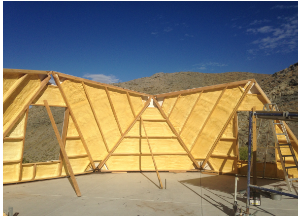
Triangular wall panels fit together to form an incredibly strong structure.
