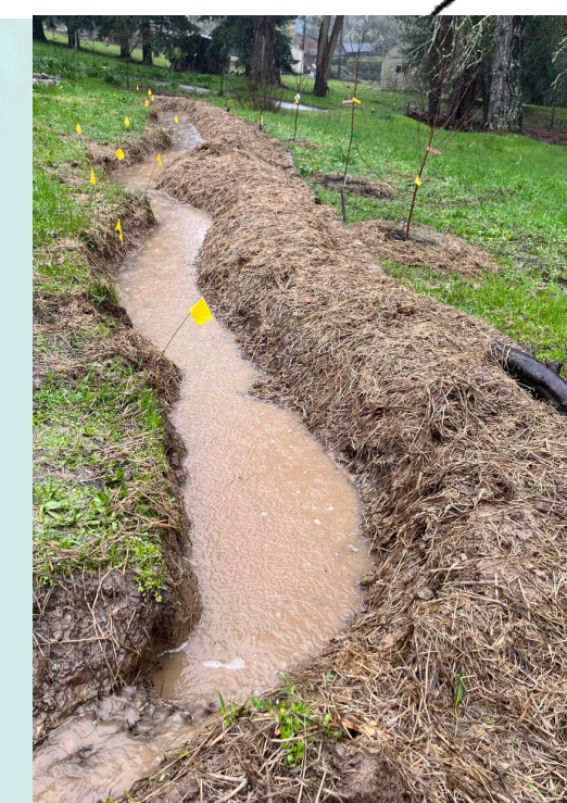
SWALES ALONG NATURAL CONTOUR LINES FOR FLOODING PREVENTION
