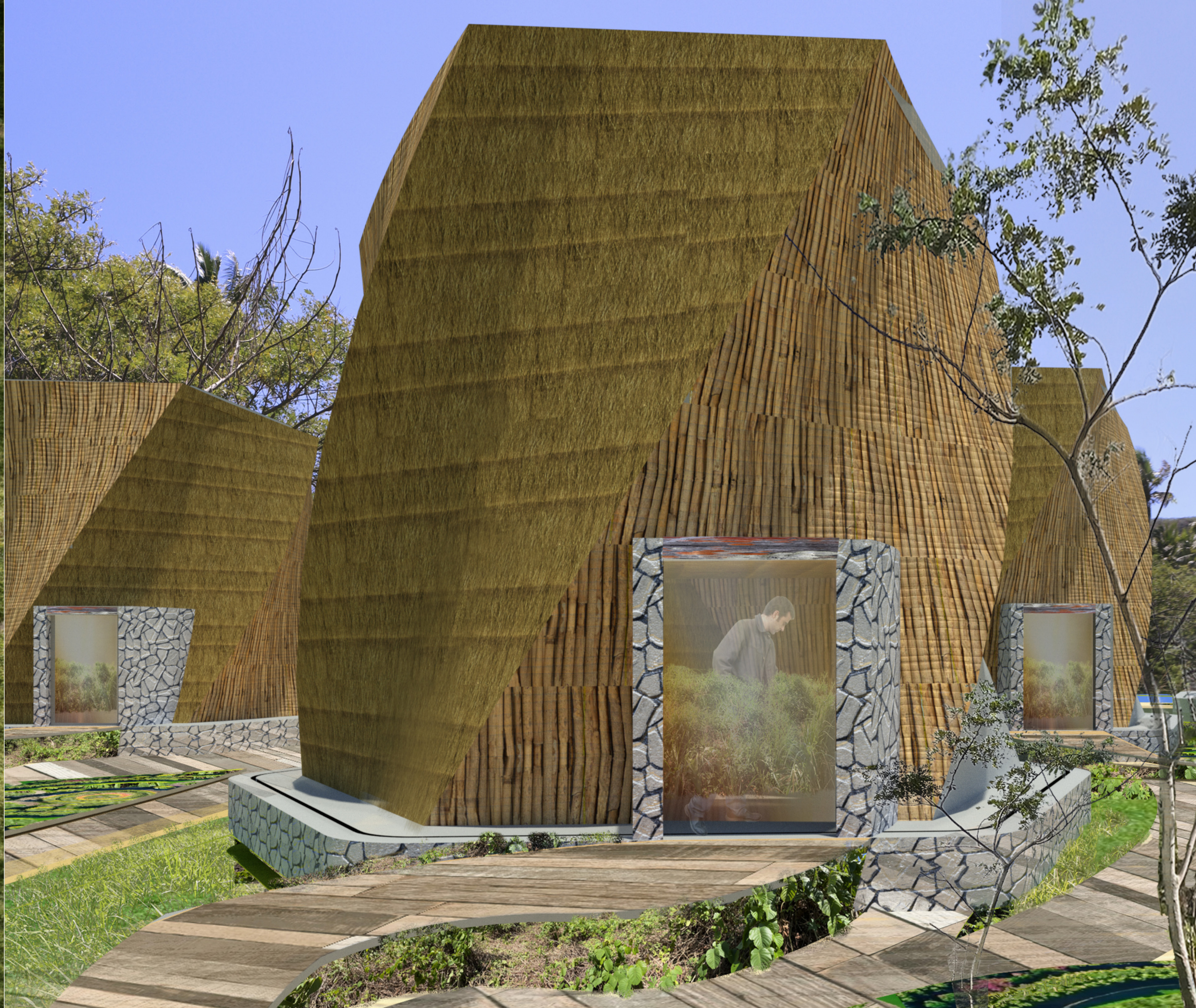
The image presents an architectural module that fuses a modern structure with local natural materials, creating a dialogue between engineering and tradition. The structural base of the module is constructed of stainless steel, providing strength and durability. This structure is clad externally in palm and bamboo, generating an organic texture and a visual connection to Naviti's tropical surroundings. Access to the module is defined by rustic stone walls and a natural wood roof, harmoniously integrating with the surrounding pathways. Gentle ramps connect the walkways to the entrance, facilitating accessibility. Through the doors, dim or semi-dark light is perceived, suggesting an interior designed for the cultivation of plants that thrive in partial shade. This module exemplifies the project philosophy by combining the solidity of a stainless steel structure with the warmth and sustainability of natural materials, reflecting inspiration from natural forms and the cultural relevance of the surroundings.
