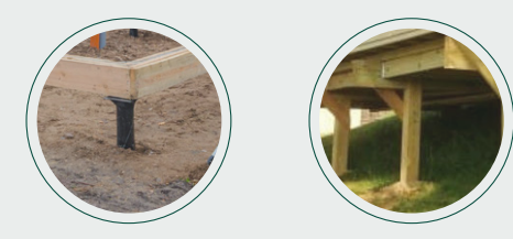
Steel Screw Pile Foundation (punctual concrete can be alternative depending on soil conditions)
