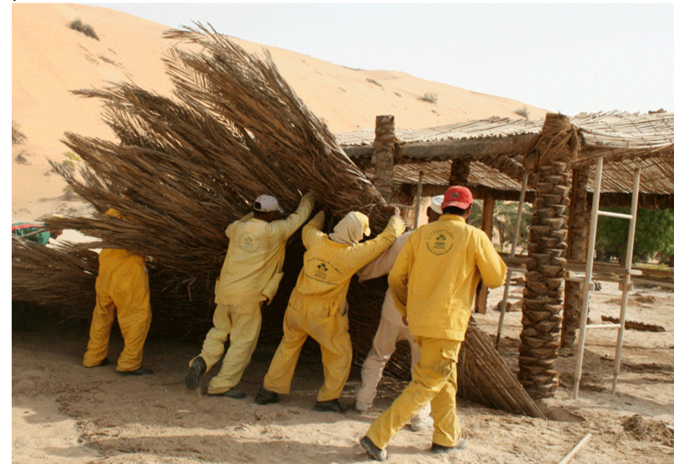
palm tree - structure
