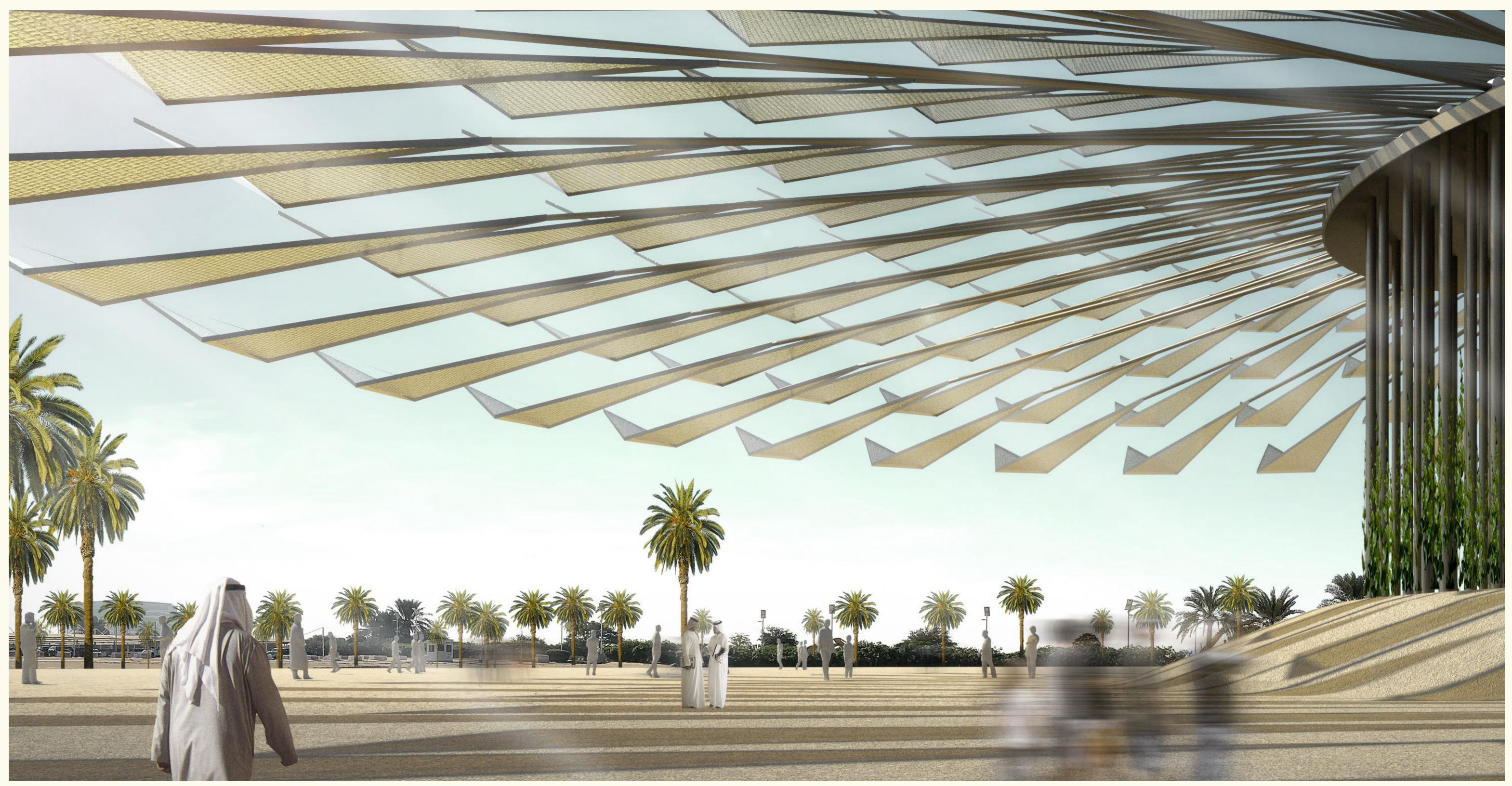
During day time, the fully open petals collect energy from the sun through translucent photovoltaic panels while providing a comfortable shade for visitors.
