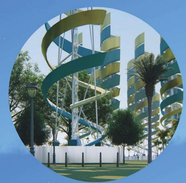
The main structure comprises of stain-less steel beams anchored in a reinforced base with foundations in the ground part of the site. The spinning skins are full lighting color which can be in different colors during days and nights.
